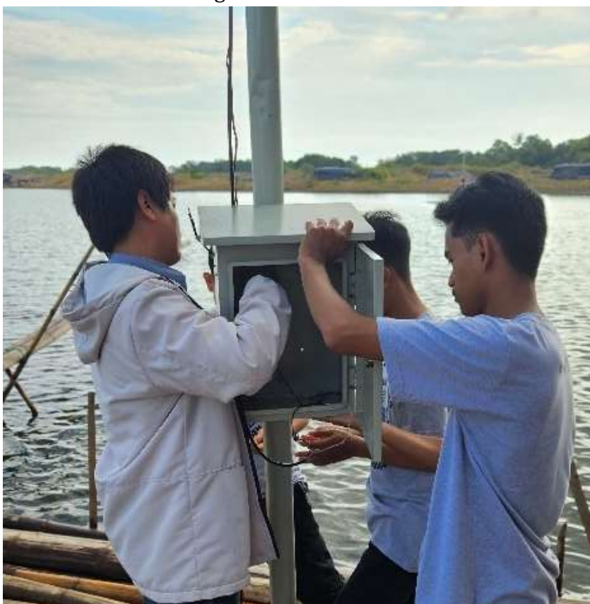
Gambar 3. Proses Instalasi Unit Monitoring Kualitas Air Bertenaga Surya
