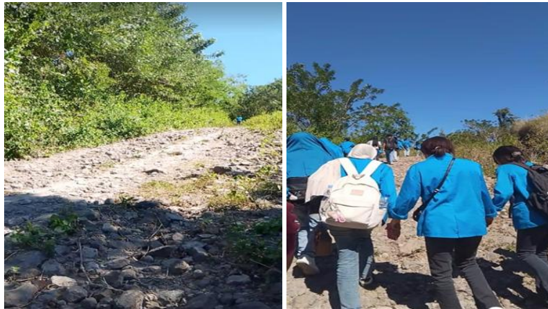
Figure 3: The condition of the road to Kawa Village and visitors walking toward the destination.
