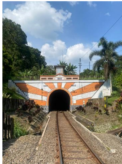
Figure 1. Mrawan BH 152A tunnel
