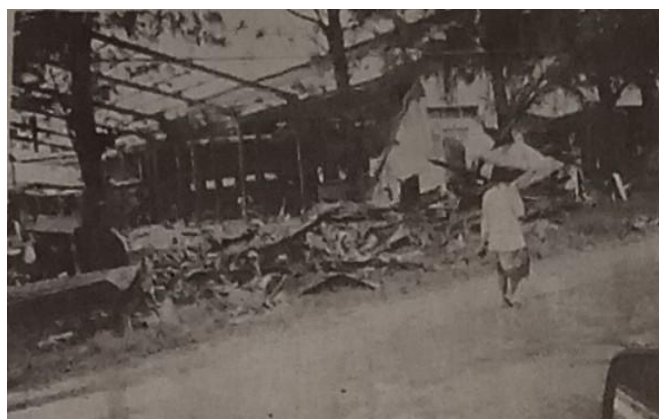
Figure 1. Damage to the Damaitex Factory Resulting from the Flood Surges (KARTIKA, 1990).
