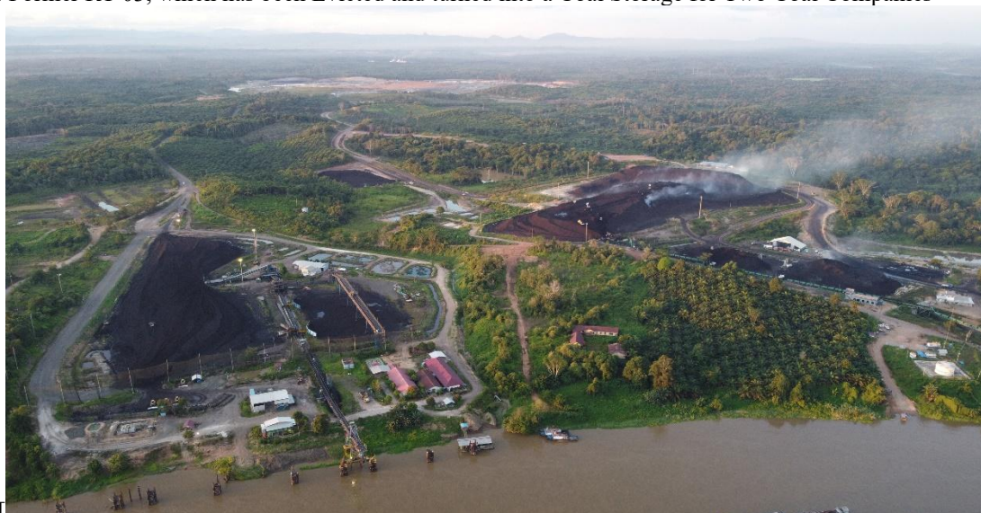
Figure 1: Former RT 03, which has been Evicted and turned into a Coal Storage for Two Coal Companies
