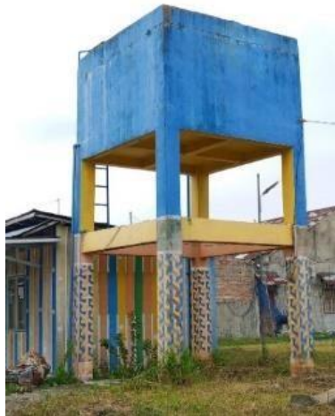
Figure 2. SPAM building in Pasar Ilalang Hamlet
